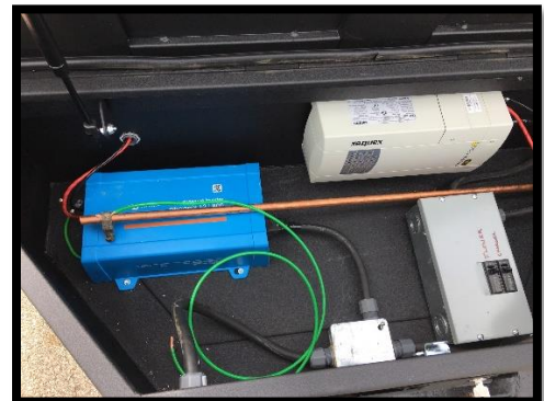
Battery charger, inverter and GND rod
