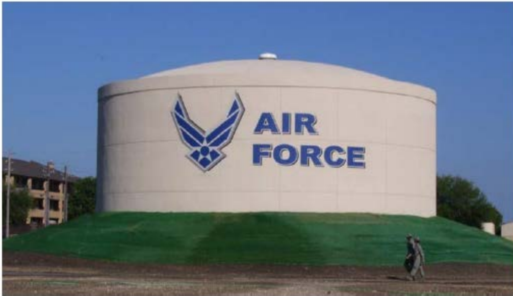
Existing Thermal Energy Storage tank at Lackland.
