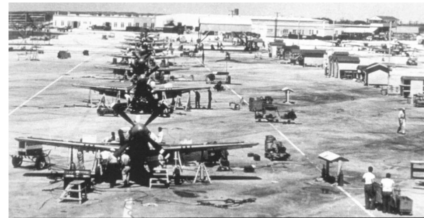
Kelly workers repairing P-51s during World War II
