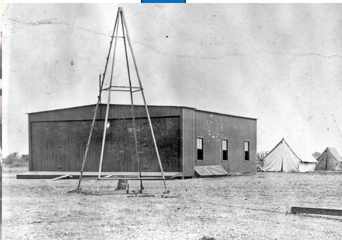
Hangar for Army Aircraft #1 on the cavalry drill ground east of New Braunfels Avenue
